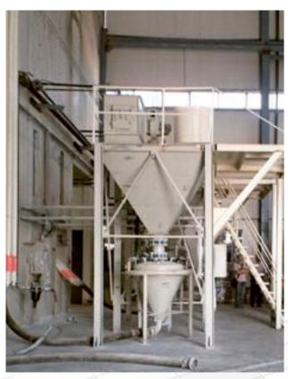
DENSE PHASE is a system in which the product is transferred in the pipe faster and denser than other systems. Used transfer air is more pressurized.
